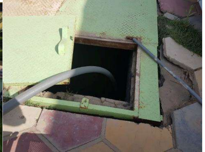
Underground concrete water tanks for saving rain waters
